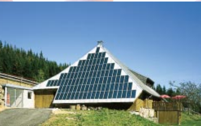
Rappenecker Hof, a Black Forest guest house which is situated far from the public utility grid. In 2003 a PEM fuel cell was installed into an existing photovoltaic/hybrid system and operates under real conditions in the guest house.
